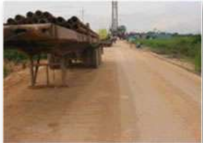
200 mm thick stabilized road floating over peat and in use after 3 months construction
